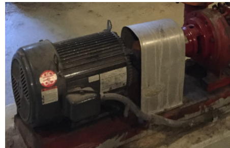
Figure 2.18: Hot water pump
