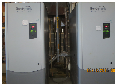
Figure 2.17: Condensing boilers
