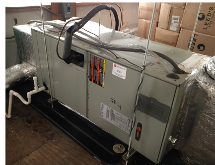
Figure 2.12: Office area Trane heat pump
