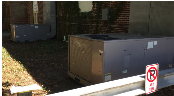
Figure 2.3: Carrier RTUs
