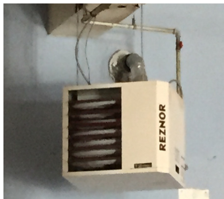
Figure 2.2: Unit Heater
