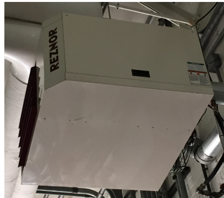
Figure 2.6: Reznor Unit Heater
