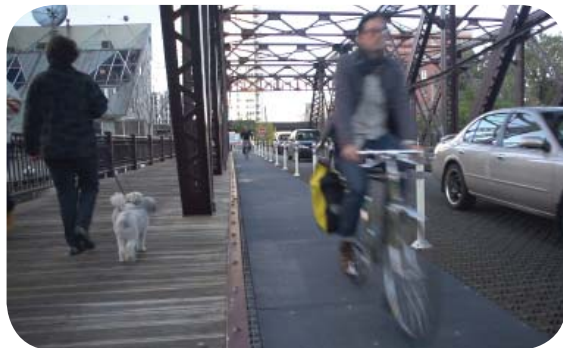
EXAMPLE OF STEEL OVERLAY
