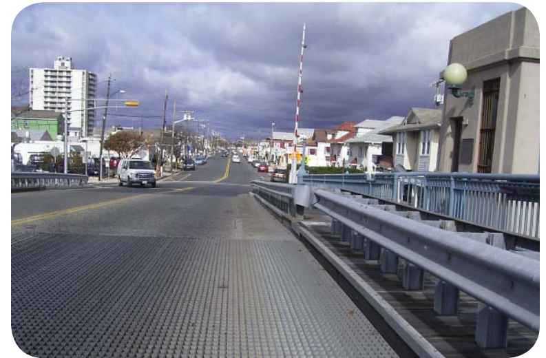
DORSET AVENUE BRIDGE
