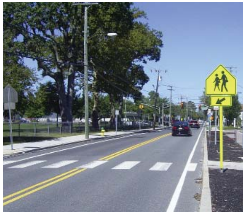
HIGH-VISIBILITY CROSSWALK WITH PEDESTRIAN WARNING SIGN
