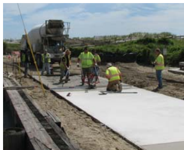
BEACH PATH CONSTRUCTION IN N. WILDWOOD
